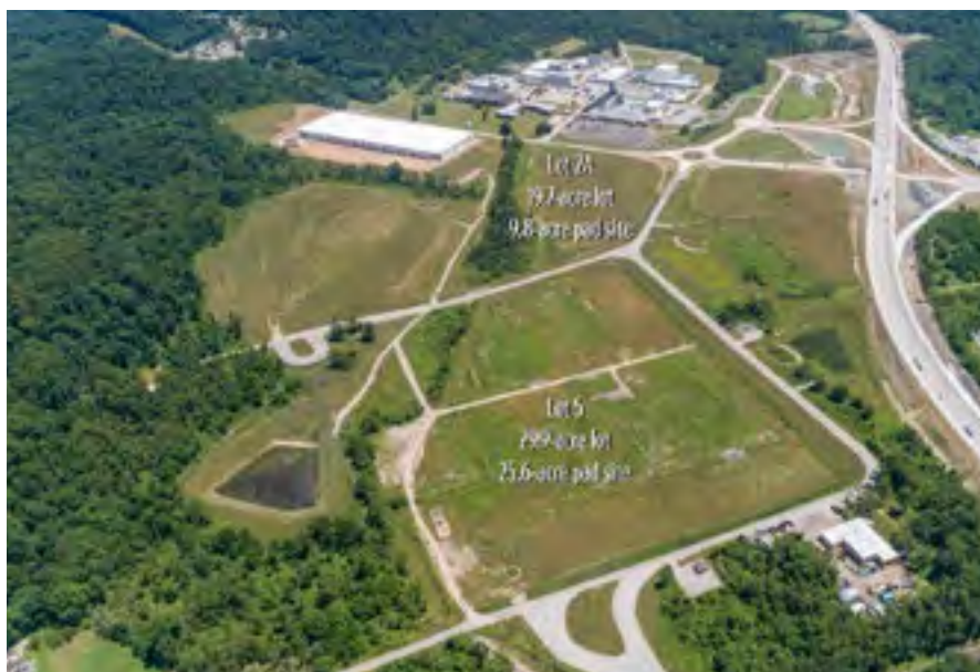
Image shows details about available pad-ready sites at Commerce Crossing at Westmoreland, PA.
